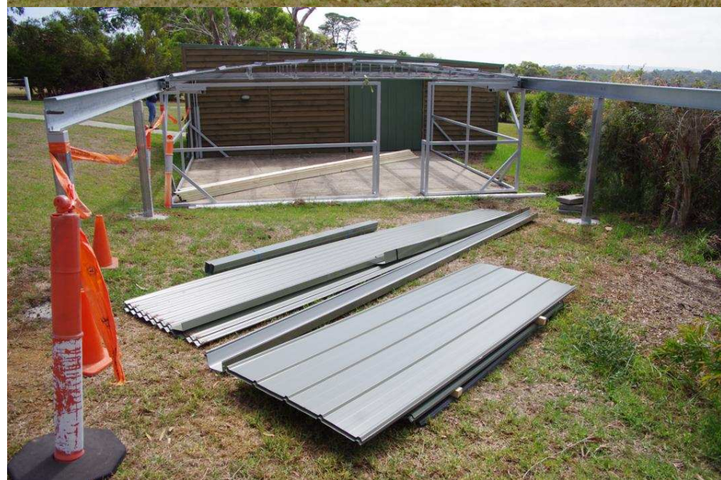
Above - The temporary wooden supports removed & the roof is on the move. We have fitted end stops in the "C" beam, so the roof can't be pushed out on to the ground.
