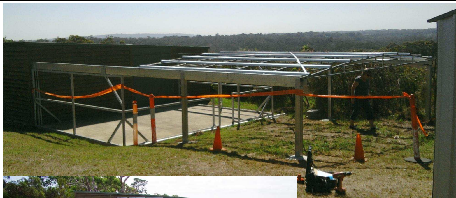
Above - The temporary wooden supports removed & the roof is on the move. We have fitted end stops in the "C" beam, so the roof can't be pushed out on to the ground.
