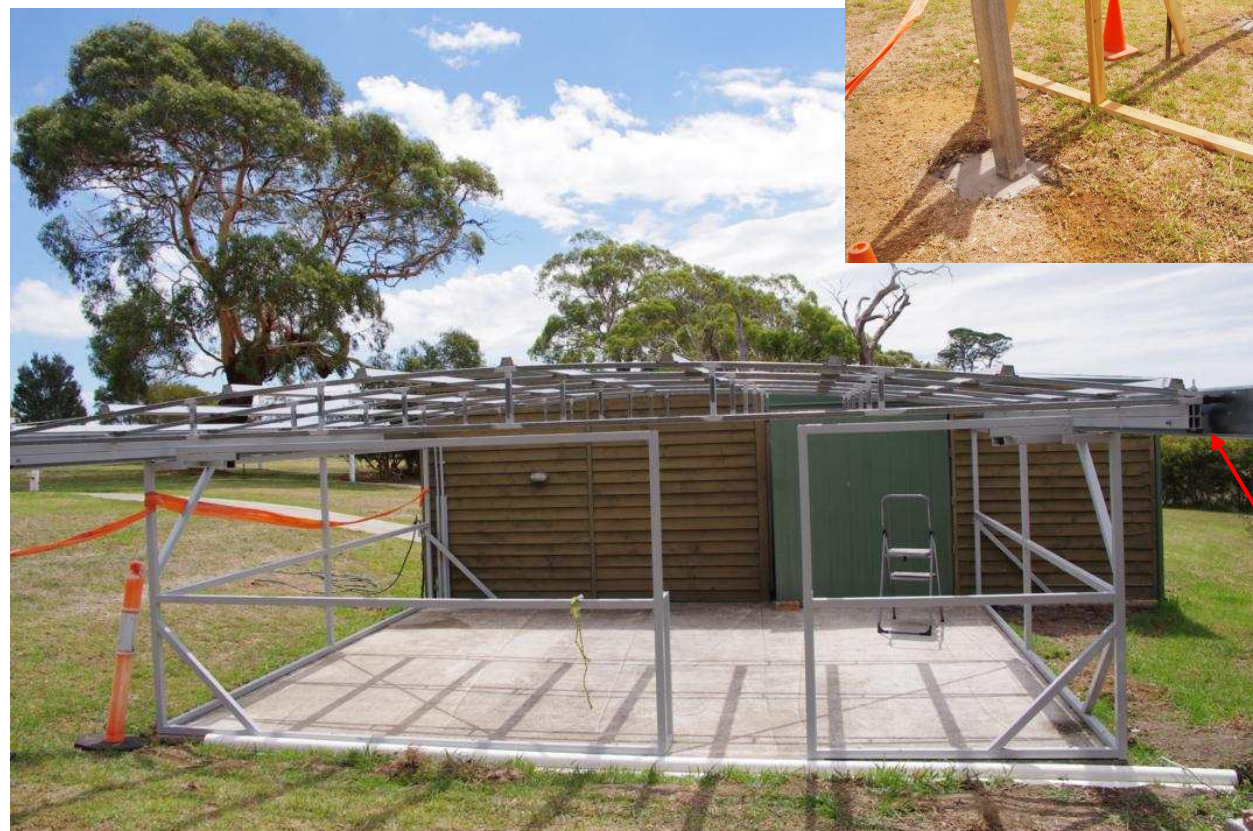
Below - close up view of wheels in "C" beam, small rubber wheel at top helps to keep the roof central & stops any metal rubbing.
